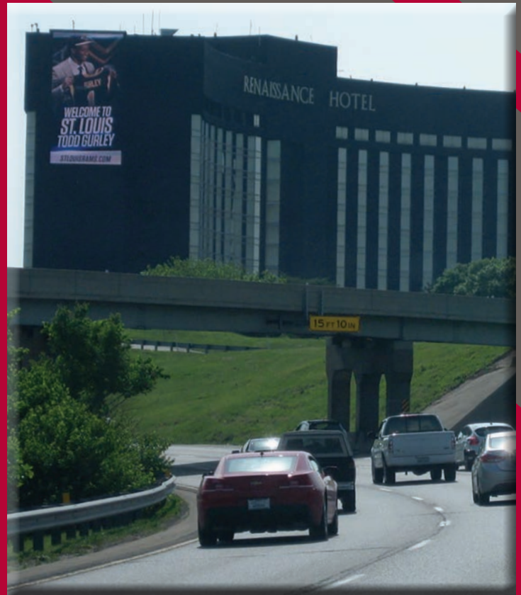
ABOVE Approach view from I-70.
